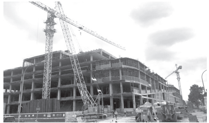
AEON shopping complex @ Jln TAZA under construction
