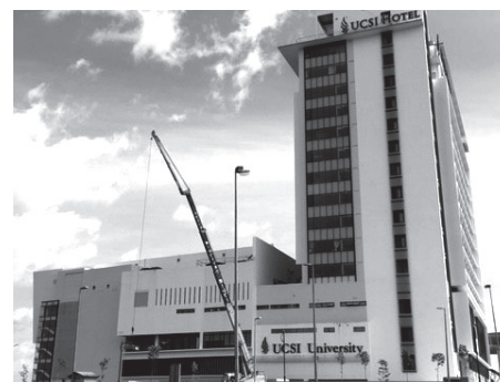
UCSI Hotel at Kuching Isthmus, nearing completion
