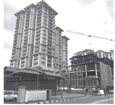
Riverine Diamond under construction at Jln Petanak
