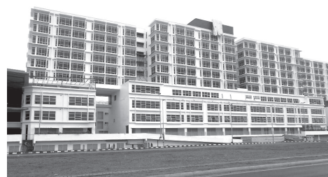
Newly completed SOVO at Bintulu Paragon
