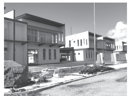
Chen Ling Factory units at Demak Laut
