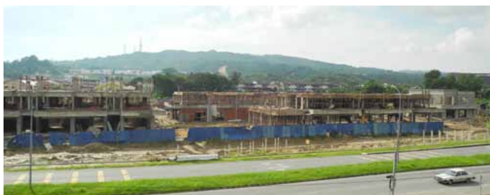
Mid - Town Project (under construction)
