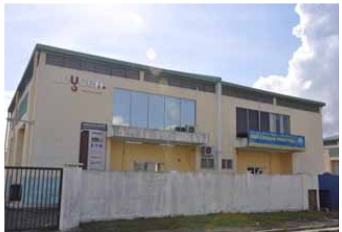
2-storey ready built factories in KKIP
