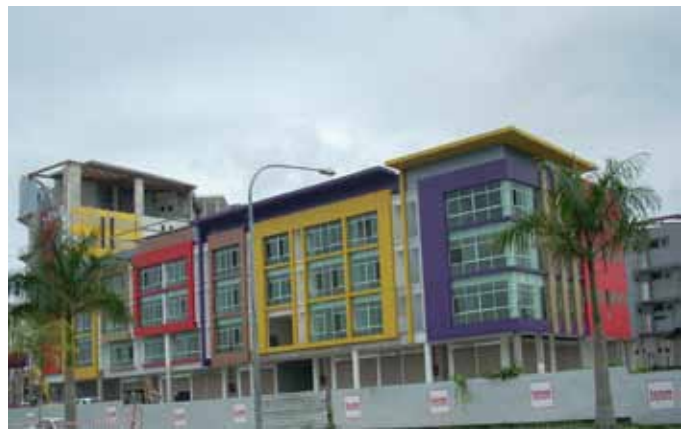
iCom Square commercial centre
