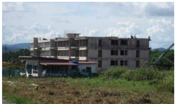
Palm Garden under construction
