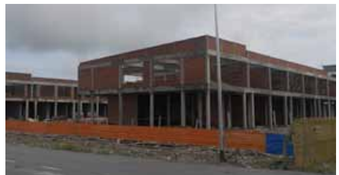
2 - storey shopoffices in Kidurong Commercial Park
