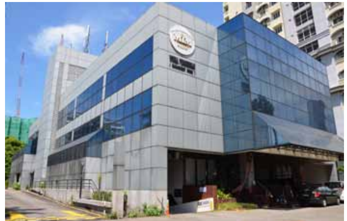
227, Jalan Ampang, KL (former MIM Building)
