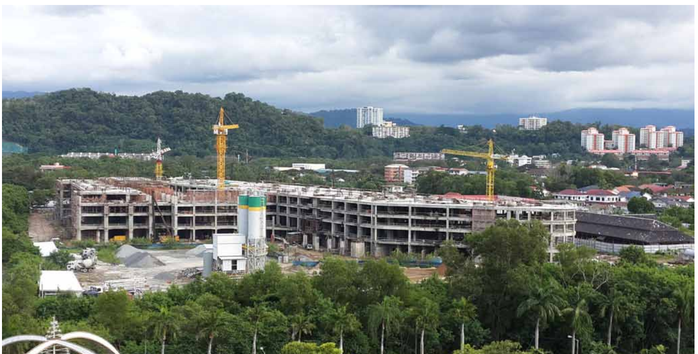
Pacific Parade Mall, under construction
