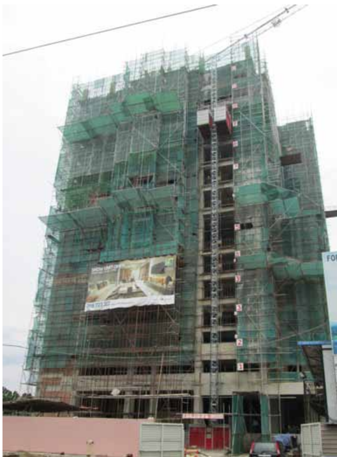
Tropicana Landmark, under construction
