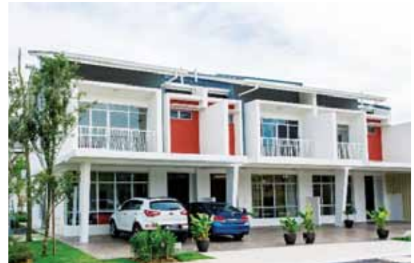
2-storey terraced houses in M Residence @ Rawang
