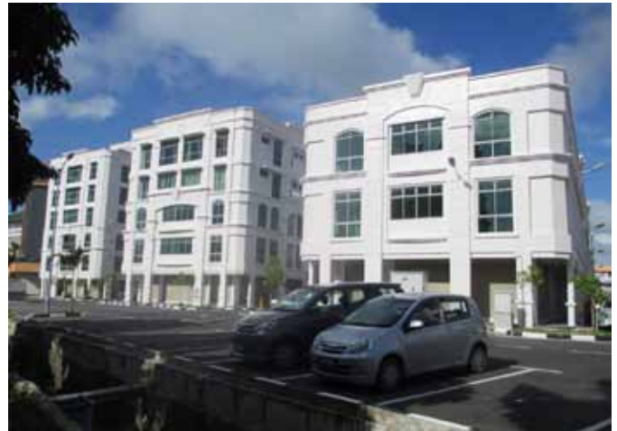
Lazenda Central shopoffices
