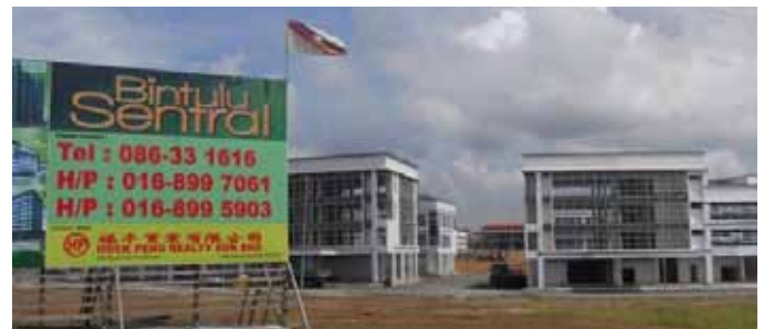
3 and 4 - storey shopoffices in Bintulu Sentral Jalan Kidurong
