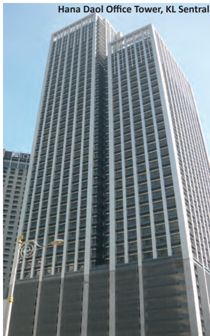
Hana Daol Office Tower, KL Sentral
