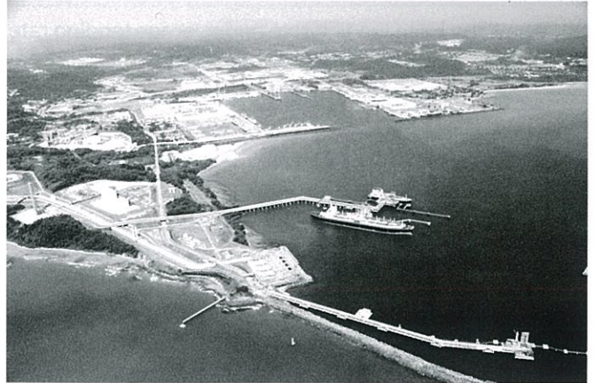
On-going extension at Bintulu Port
