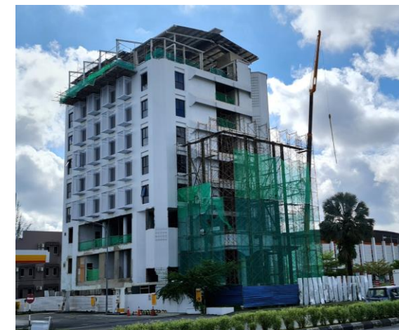
Roxy Impiana undergoing refurbishment, Kuching Source: WTWY Research
