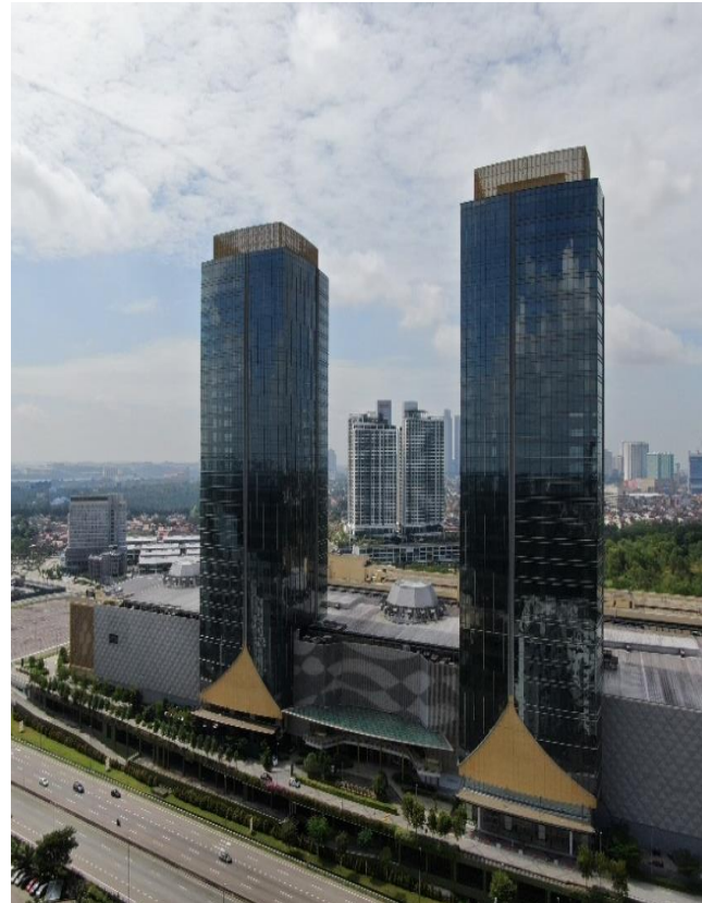
MVS South and North Towers in Midvalley Southkey, Johor Bahru Source: CBRE | WTW Research
