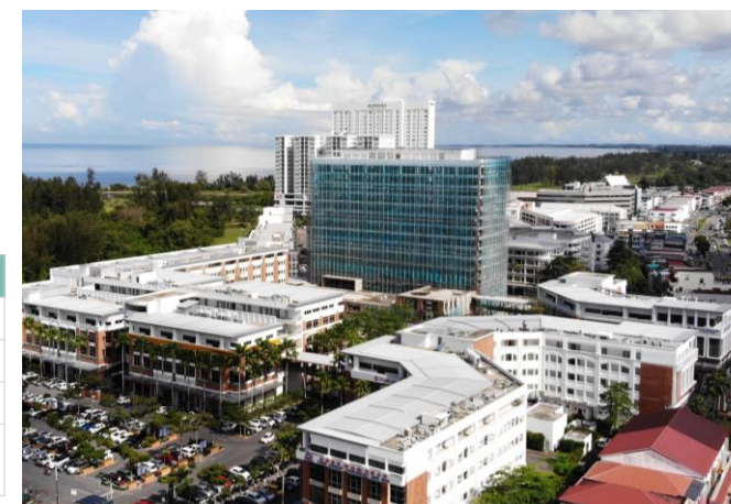
Shell Malaysia HQ Building at Miri Times Square, Marina Park City (under construction) Source: WTWY Research
