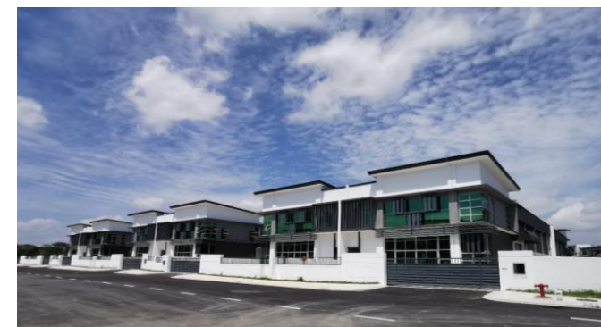
Newly Completed Factories, Kempas Utama Industrial Park Source: CBRE | WTW Research
