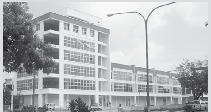
6-storey office building together with adjoining 3-storey shophouses at Jalan Pedada.
