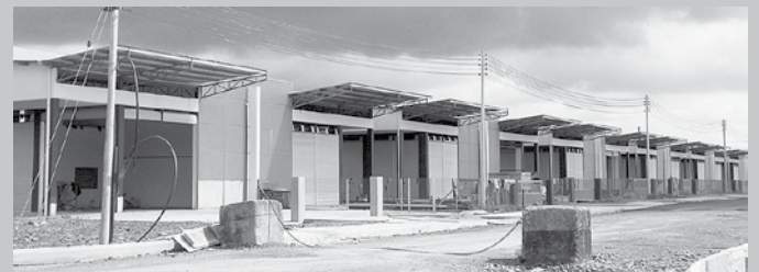
Industrial Building at Kidurong Commercial Centre
