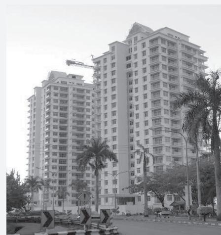
Bay Resort (nearing completion) located along Jalan Temenggong Oyong Lawai Jau, next to Taman Selera in Miri
