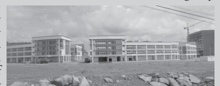
Bintulu Sentral at Jln Kidurong
