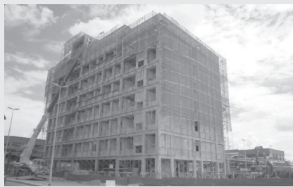
7 storey hotel under construction within Medan Jaya Commercial Centre
