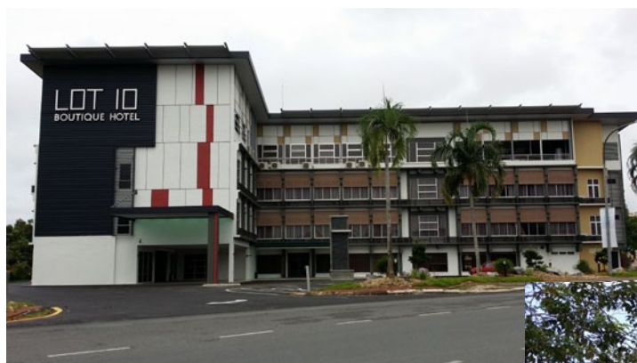
Lot 10 Boutique Hotel at Jln Ban Hock-Central Timur
