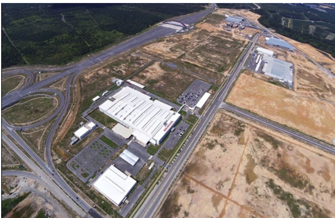
The main portion of Batu Kawan Industrial park being developed
