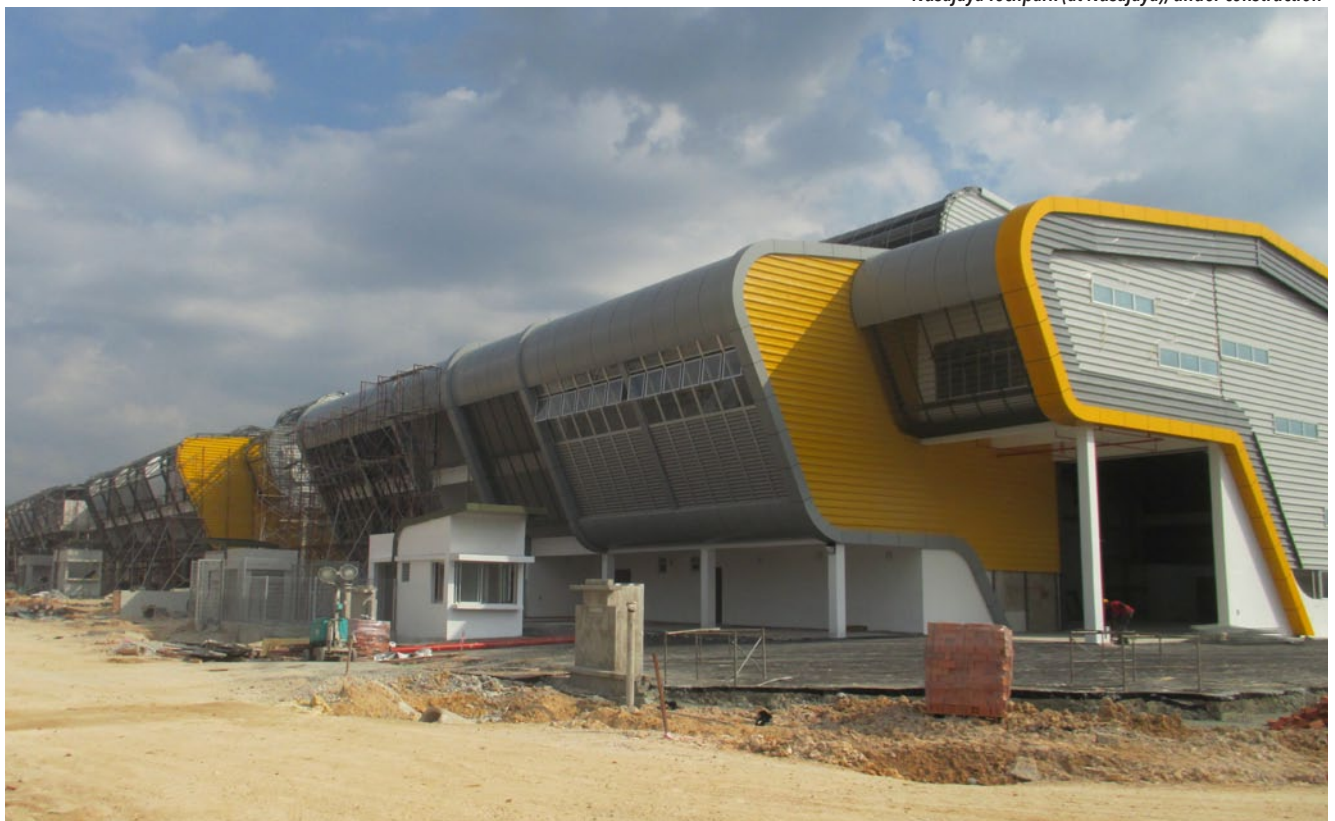
Nusajaya Techpark (at Nusajaya), under construction
