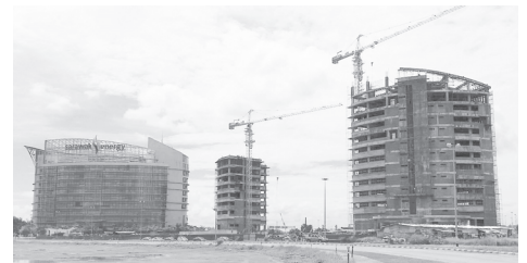
The Gateway Towers, purpose-built offices housing SEDC and LCDA Headquarters at the Kuching Ishtmus
