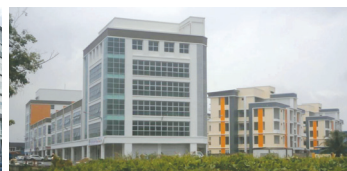
Mixed development at Lee Garden along Jalan Pedada, Sibü
