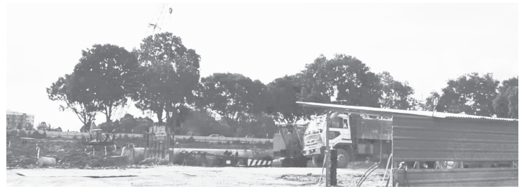
Site Clearing for AEON Shopping Mall at Jln Tun Ahmad Zaidi Adruce/ Jalan Permata, Kuching
