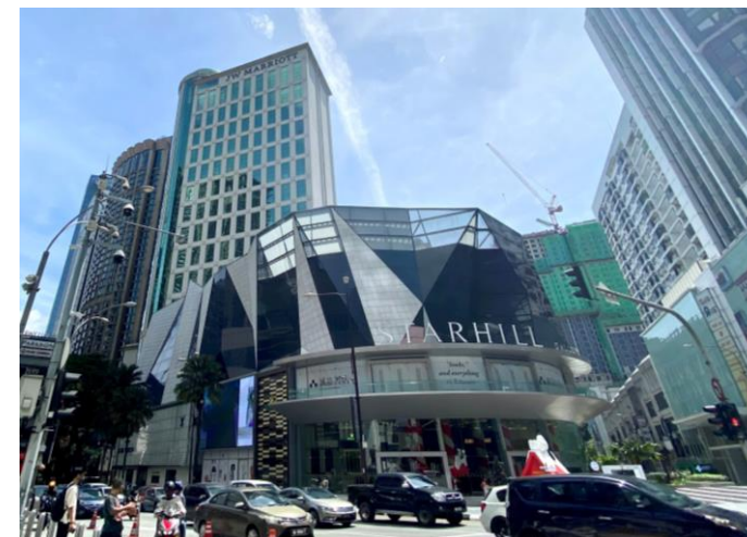
Renovated The Starhill, Bukit Bintang Source: CBRE | WTW Research
